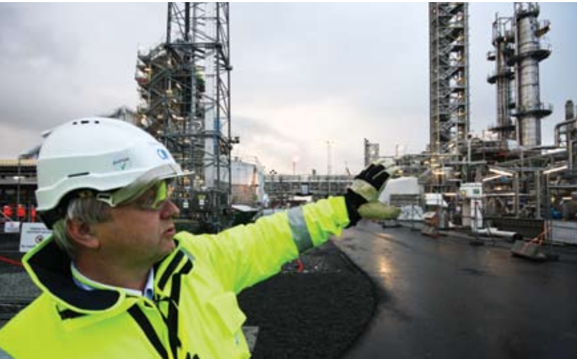
TECHNOLOGY MANAGER OLAV FALK-PEDERSEN GESTURES AT AN AMINE PLANT, ONE OF TWO TECHNOLOGIES DESIGNED TO STRIP CARBON DIOXIDE FROM POWER PLANT EXHAUST. LONG-TERM PLANS CALL FOR BUILDING A FULL-SCALE CARBON CAPTURE FACILITY AT THE SITE. AT RIGHT, THE TECHNOLOGY CENTER'S ASPIRATIONAL SLOGAN
